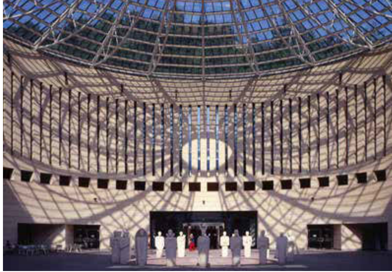
The MART museum of modern and contemporary architecture in Rovereto (Italy) - ©Enrico Cano
